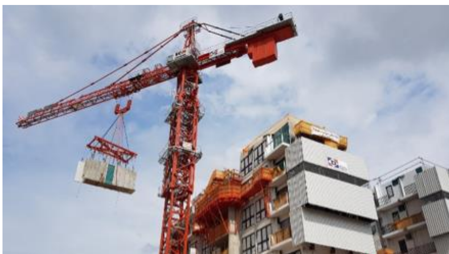
Figure 2.4. Tower Crane Hoisting of PPVC module (Seng and et al., 2021).
