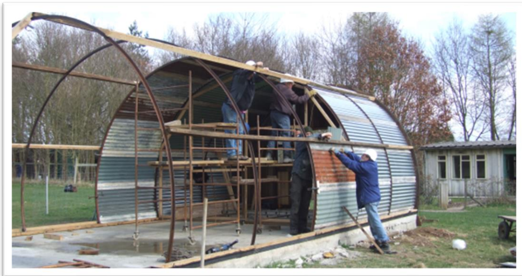
Figure 2.1. Nissen Hut under construction (College of Arms, n.d.)
