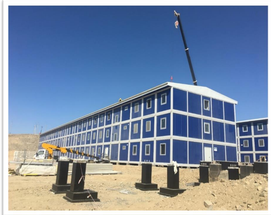
Figure 4.2. Photograph of the Aktogay Accommodation Complex
