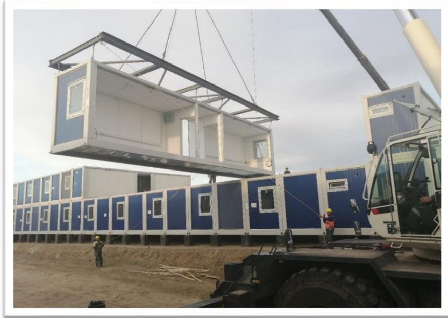
Figure 4.1. Photograph of the Aktogay Accommodation Complex
